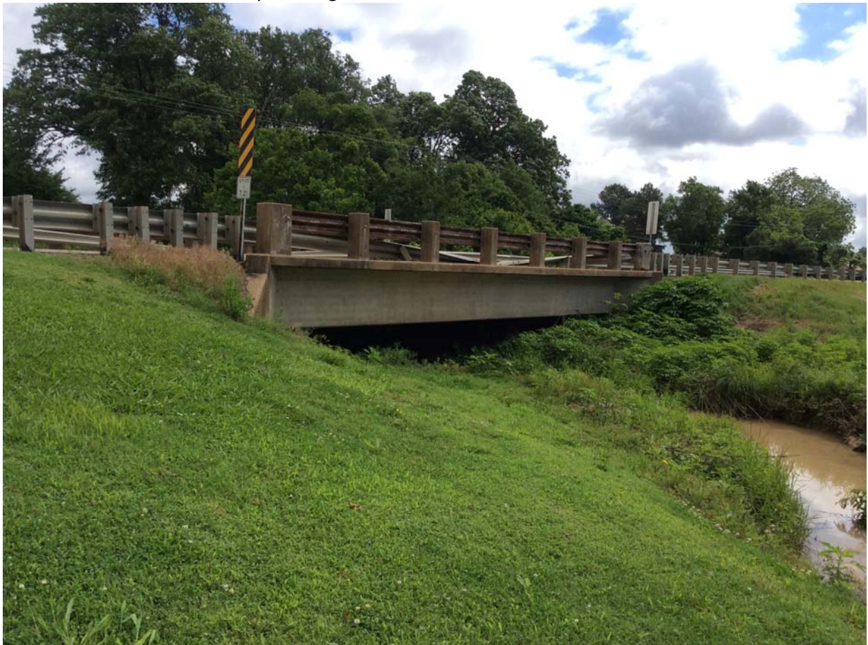
Note: 7 inches of ACHM overlay on bridge deck.
