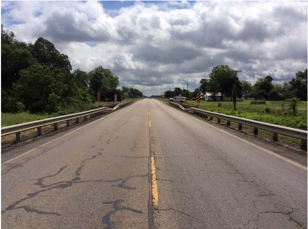
Note: 7 inches of ACHM overlay on bridge deck.
